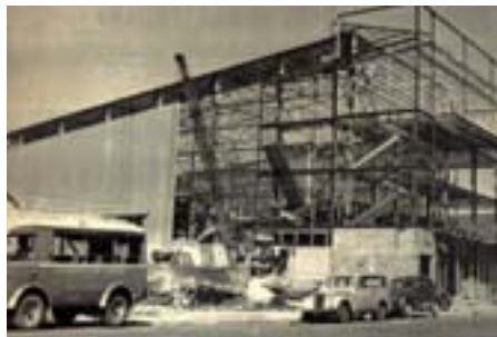
Construction du Liberty, coll. MDVN
